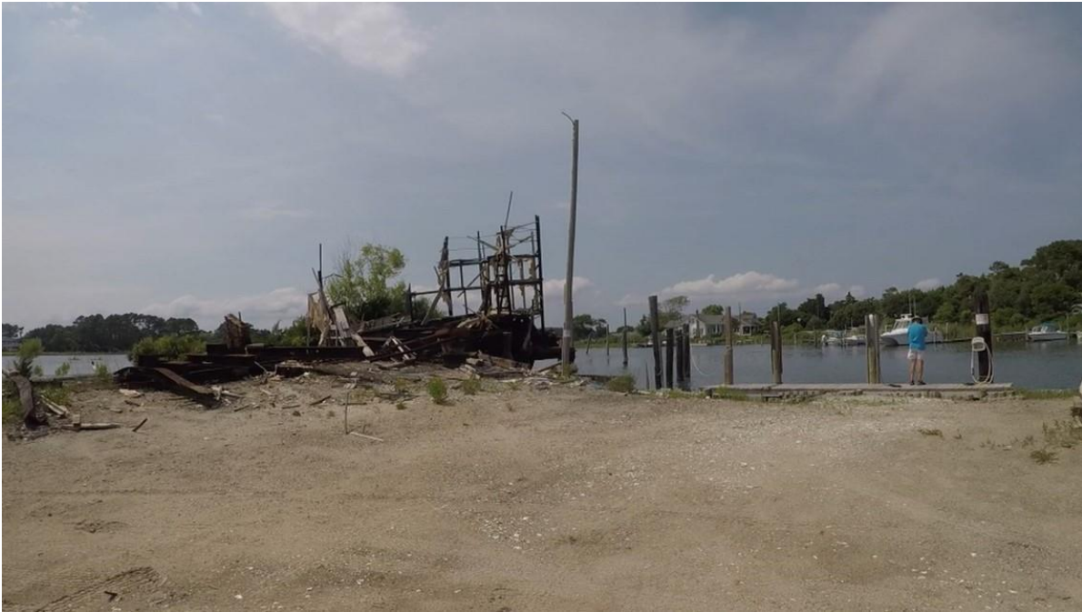
Figure 153. Abandoned dry dock boat lift apparatus (Photo by Lynn Harris, ECU).
