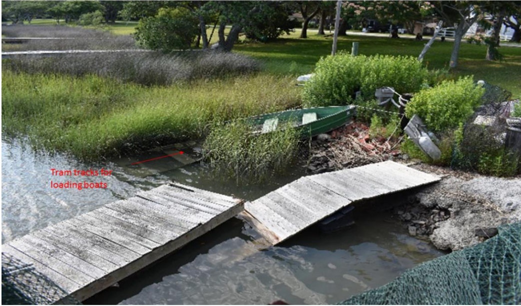
Figure 131. Old Tram Tracks for loading boats (Photo by Lynn Harris, ECU)
