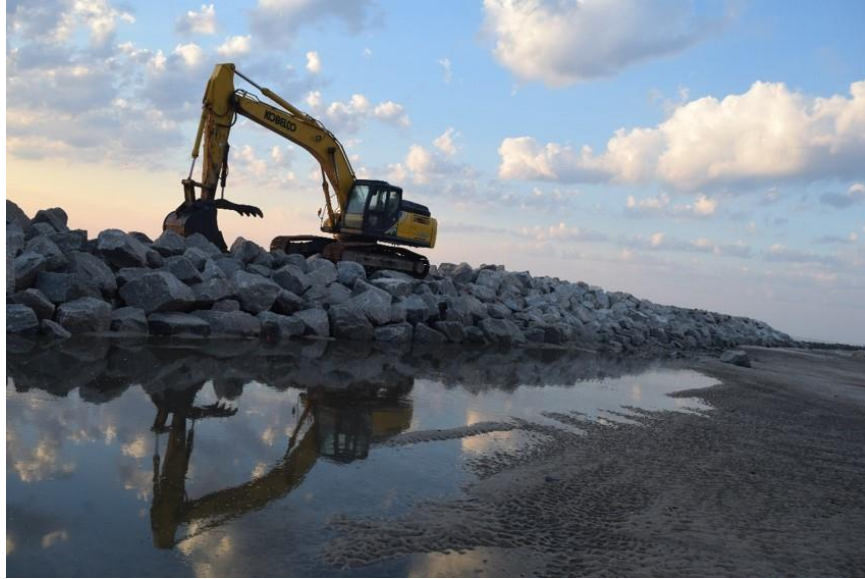
Figure 58. Rock Revetment under Construction on Driftwood beach (Photo by Jeremy Borrelli).
