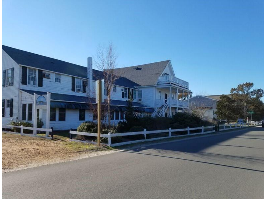
Figure 84. East Side Façade showing stairway to top rooms (Photograph by Lynn Harris, 2017)
