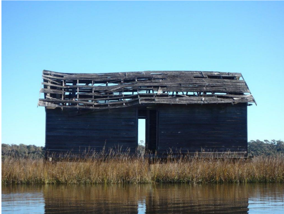
Figure 120. West face of boat house (Photo by Tyler Ball, ECU).
