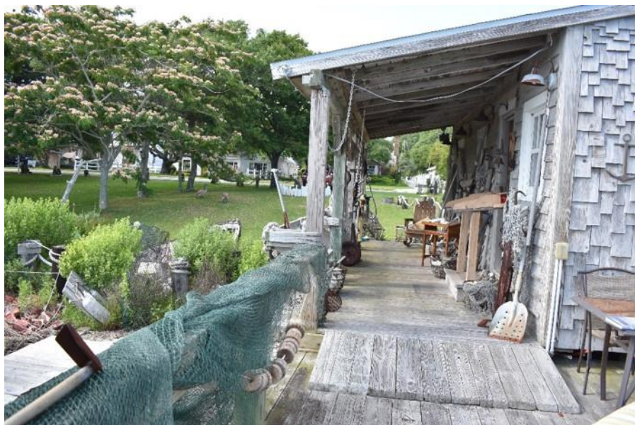
Figure 130. View of side porch from the water showing shingle construction (Photo by Lynn Harris, ECU)
