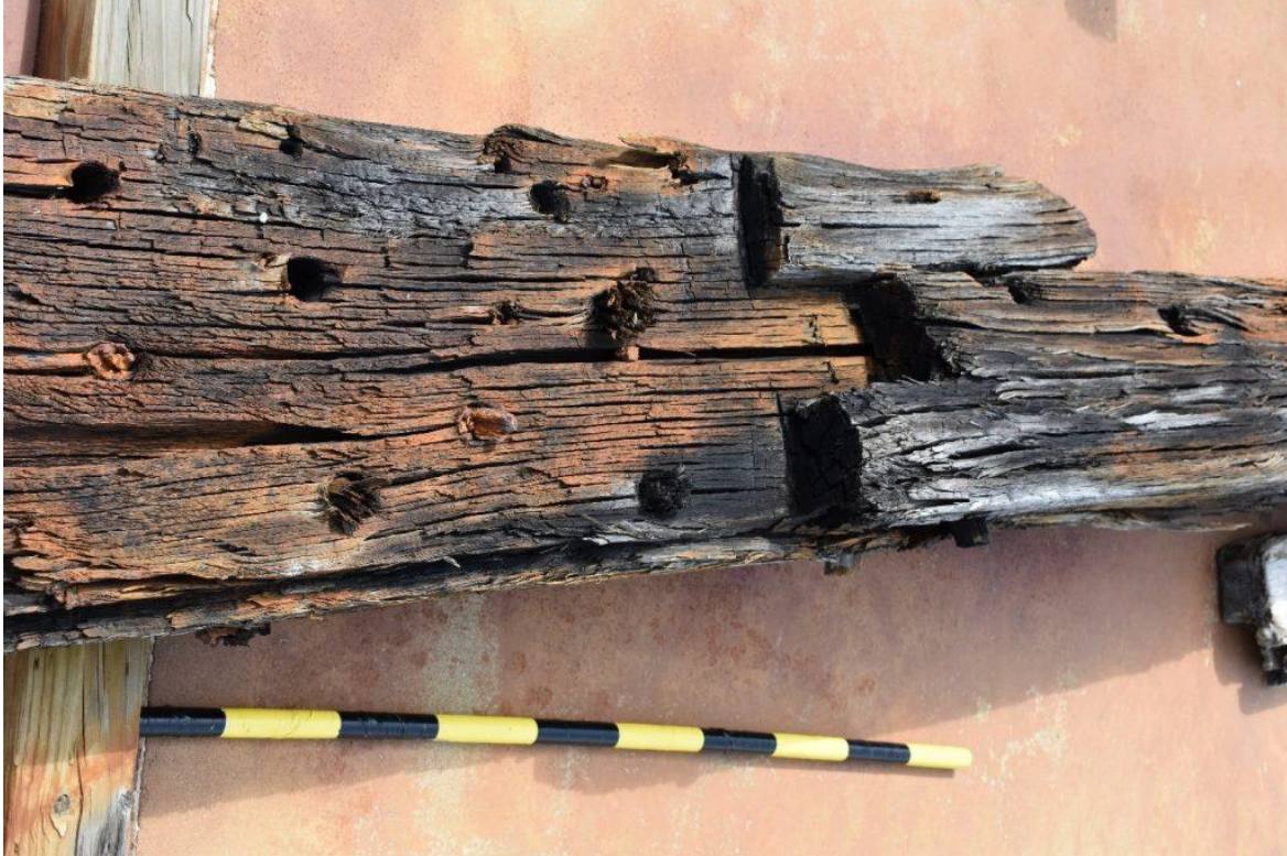
Figure 28. Rust stains on timber (Photographer Tyler Ball, ECU)
