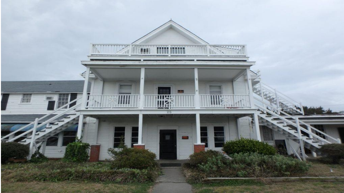
Figure 86. Front North façade showing room balconies (Photograph by Lynn Harris, 2017)
