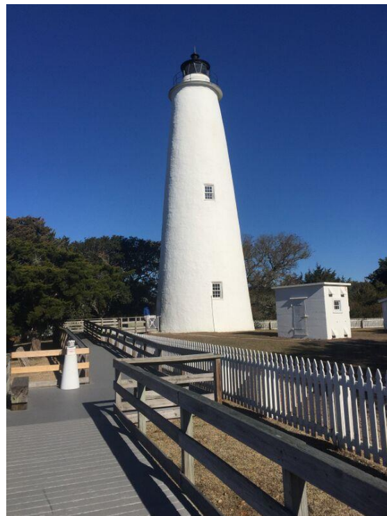
Figure . Deck constructed for public viewing of the lighthouse.
