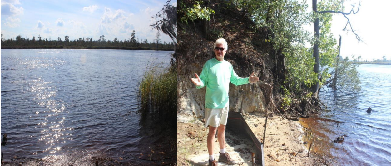
Figure 21. Boat Ramp in progress that may impact the shipwreck site with boat traffic and wake (Photo Lynn Harris)
