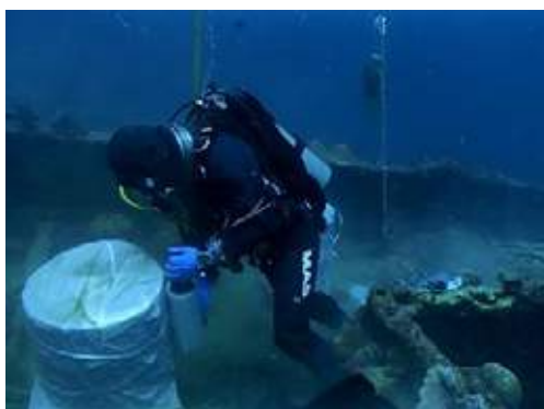
g. Charge covered with plastic wrap
