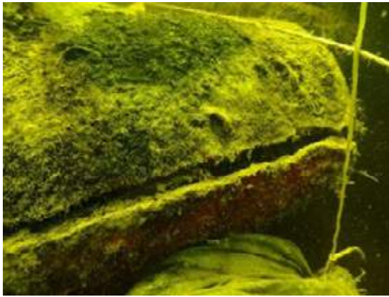
a. Crack along the welding seam
