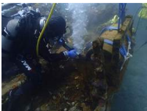
e. Removal work with an air saw
