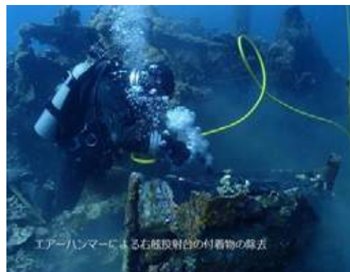
b. Coral cleaning with an air hammer drill
