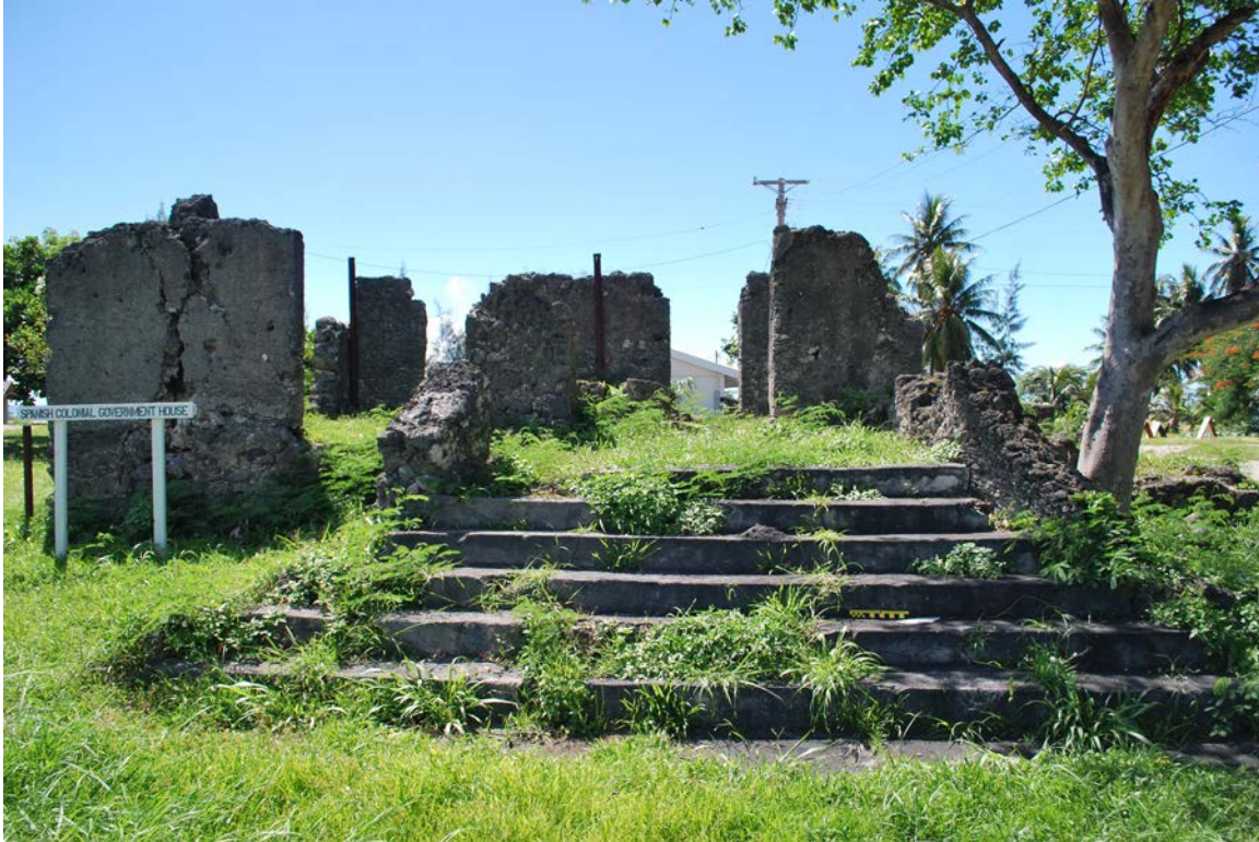
Figure 2. The Spanish government building located on Rota (J. McKinnon).
